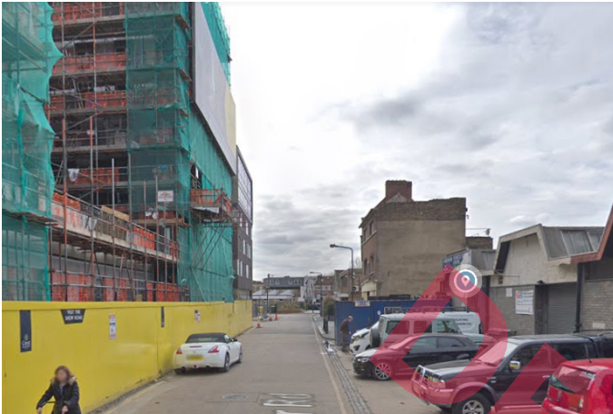
Key View 01: Brunner Road looking west
